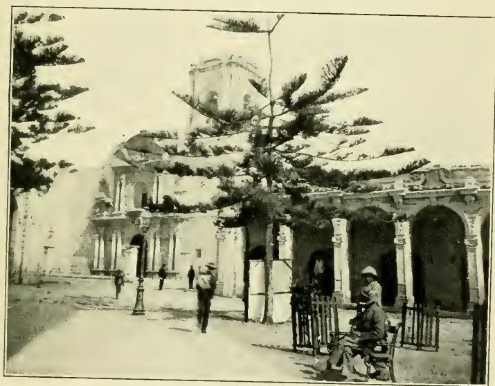
AREQUIPA CATHEDRAL TOWERS
